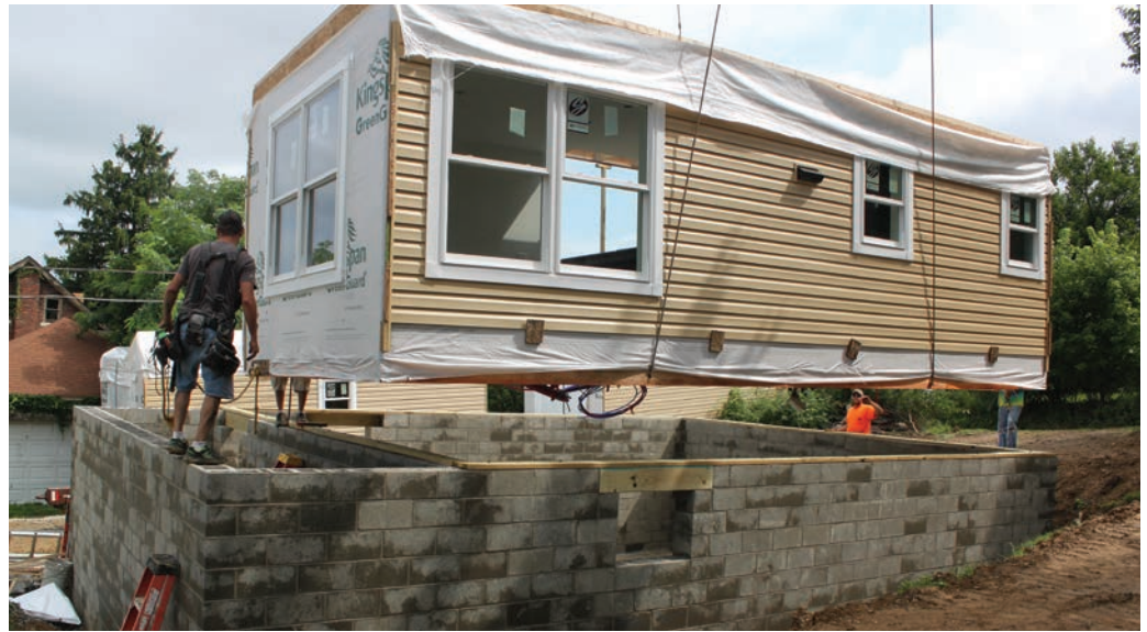
In addition to rehabilitating older buildings, MVI also constructs new housing in the communities it serves. In July 2017, crews from Structural Modulares Inc. of Clarion County and Disaster Restoration Services of Pittsburgh completed a new three-bedroom, two-story single-family home on Graham Avenue in Monessen. The house replaced an older frame house that was demolished due to mine subsidence.
